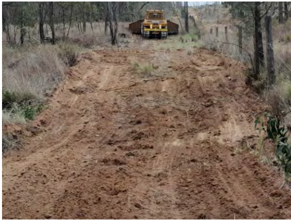
Figure 9-3 Graded access track / fire break
