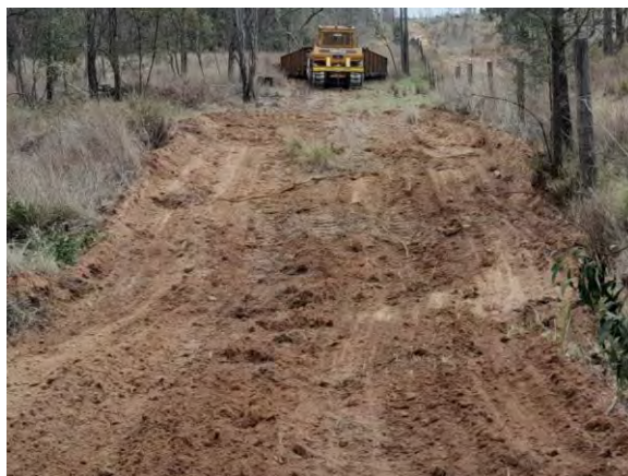
Figure 8-1 Graded access track / fire break
