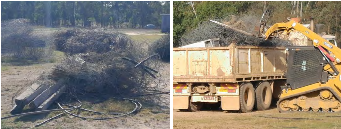
Figure 7-1 Internal removal conducted in September 2024 (left: removal from offset area, right: removal from Property)
