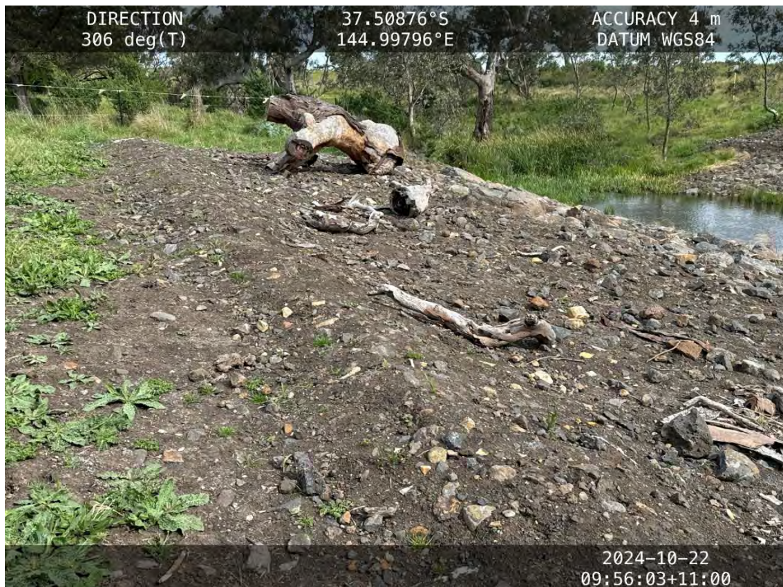
KP 42 Merri Creek – diversion berm along the bank with minimal vegetation growth and bank stabilisation evident.
