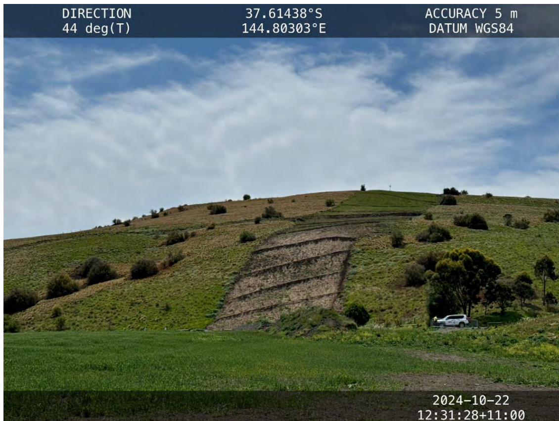
KP 16.8 Deep Creek – revegetated pasture with view of slope rehabilitation.
