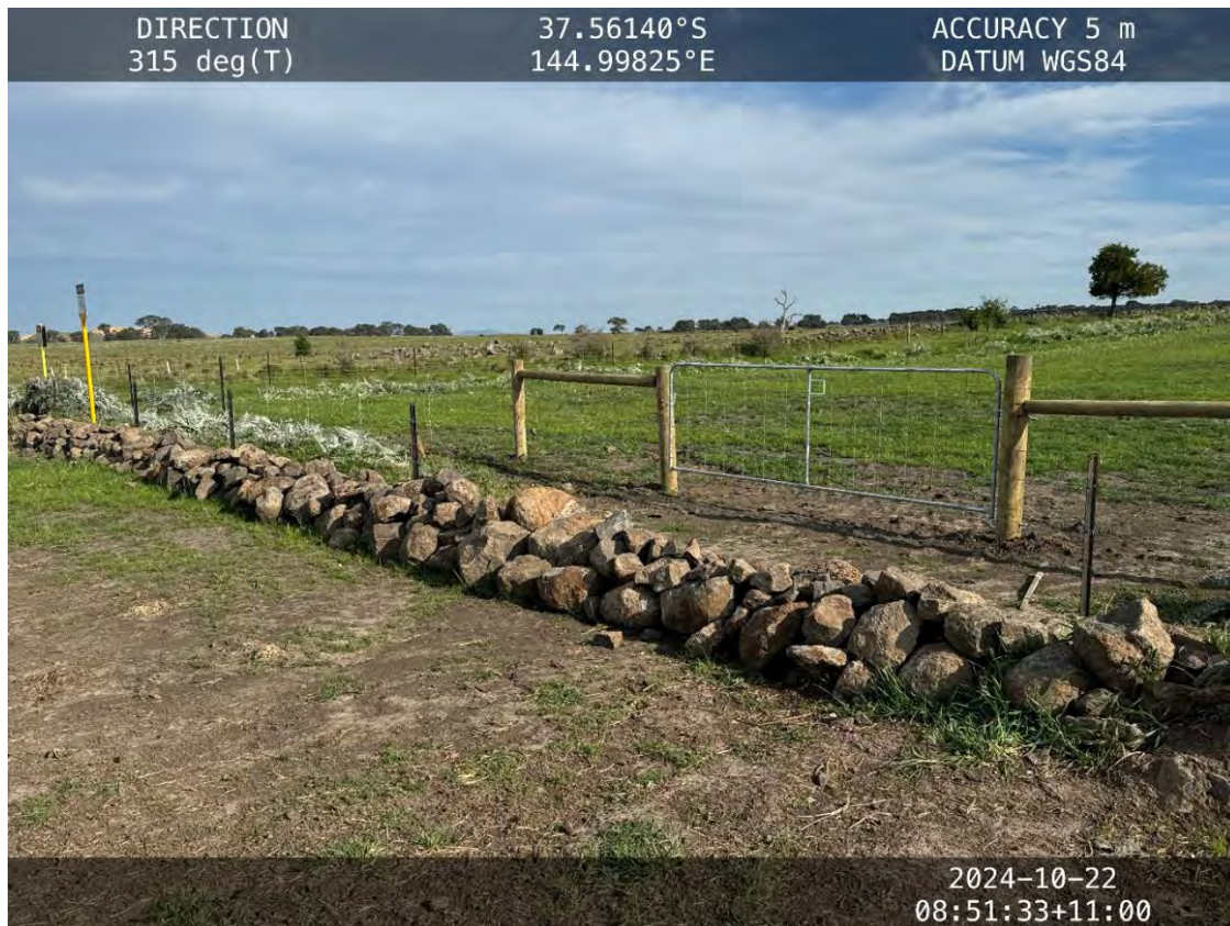
KP48.6 Conservation area 28b – reinstated rock wall across the rehabilitated pipeline right of way, stable ground with minimal vegetation growth.
