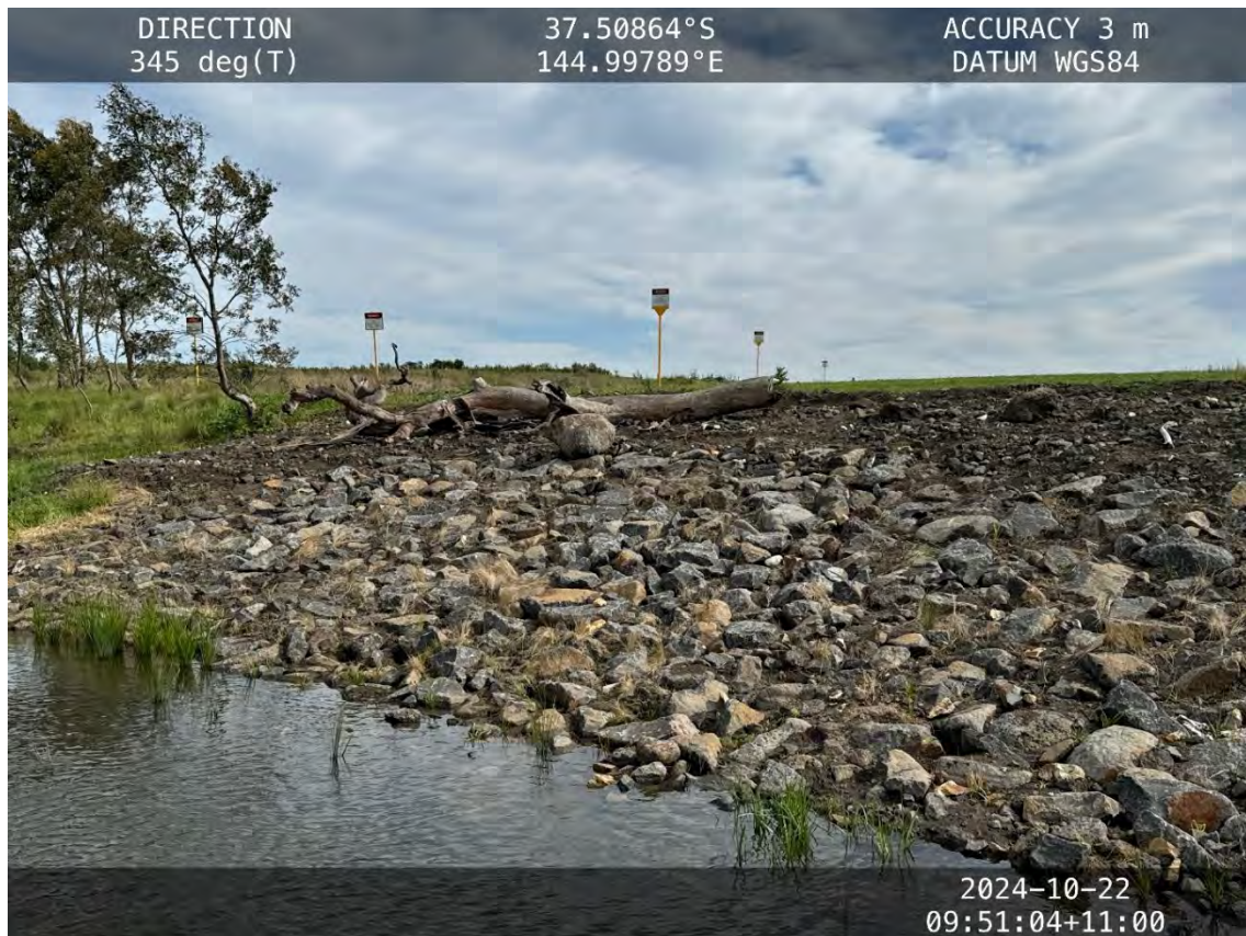
KP 42 Merri Creek – northern bank stabilisation with tubestock growth and tree placement
