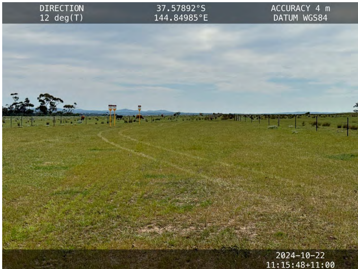
KP 22.6 to 22.8 Property 1 PS733045 – rehabilitated pipeline right-of-way and pipeline markers.
