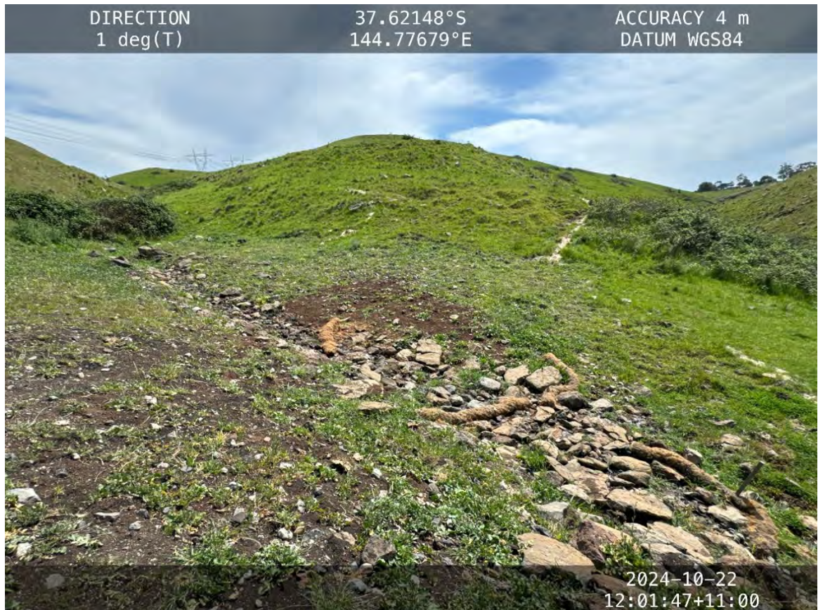
KP 13.8-14 Jackson Creek – degrading coir logs to control erosion.
