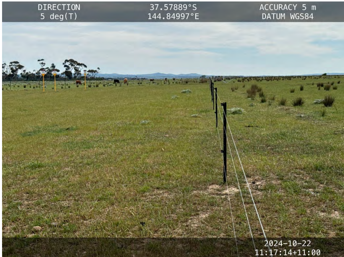
KP 22.6 to 22.8 Property 1 PS733045 – installed fence and vegetation matching the surrounding area.
