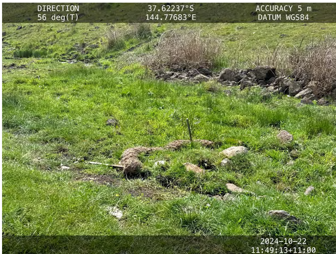
KP 13.8-14 Jackson Creek – degrading coir logs used to control erosion at the emergency work area.
