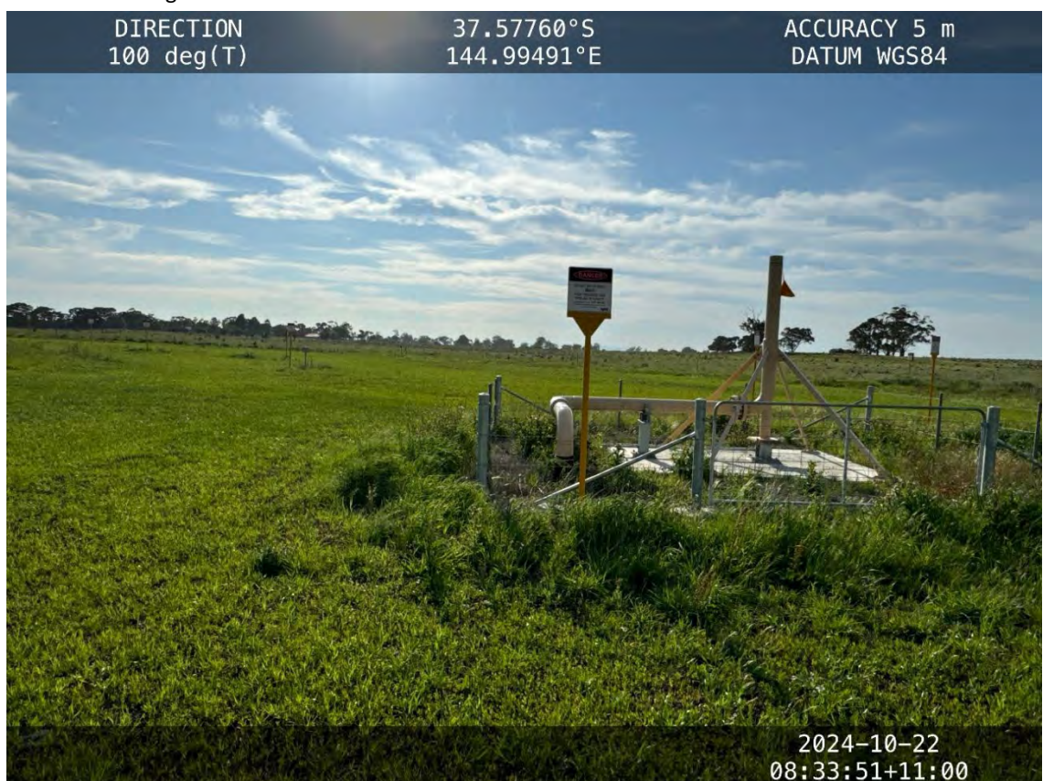
KP50 Wollert Compressor Station – vegetation coverage surrounding pipeline facility.
