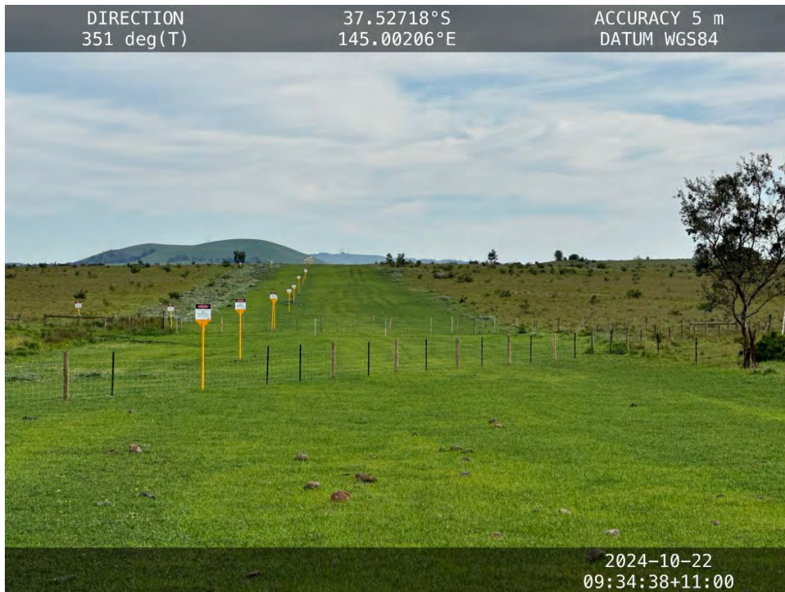
North of Donnybrook Road (adjacent to new residential area) – rehabilitated RoW with fencing and pipeline markers installed.
