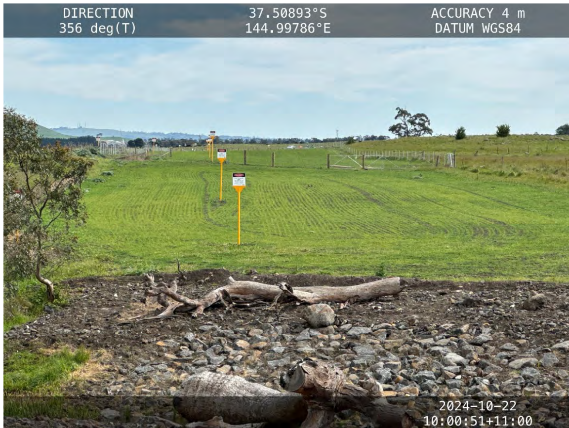
KP 42 Merri Creek – north bank with vegetation growth and pipeline markers.
