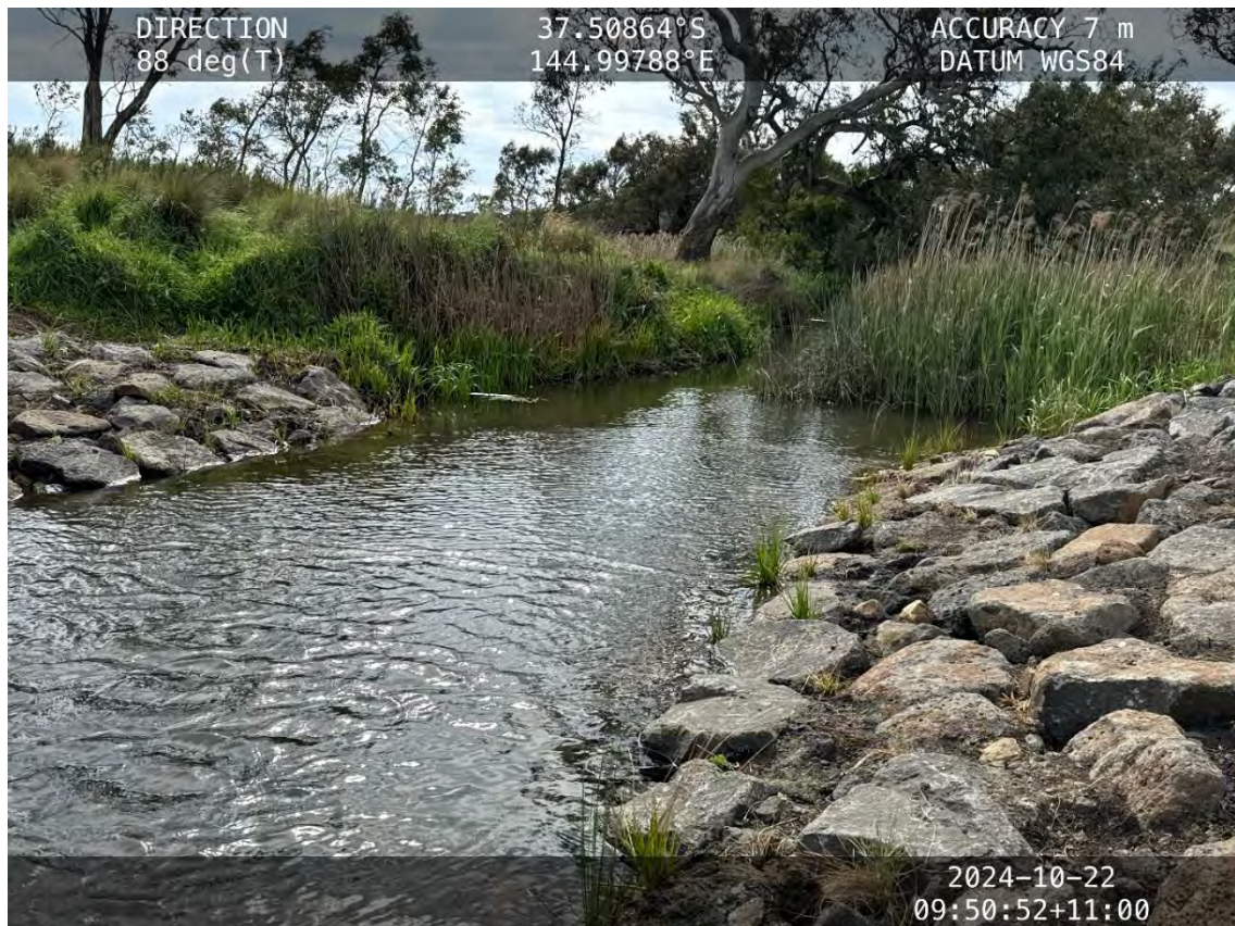
KP 42 Merri Creek – downstream view with water movement through the right-of-way and bank stabilisation.
