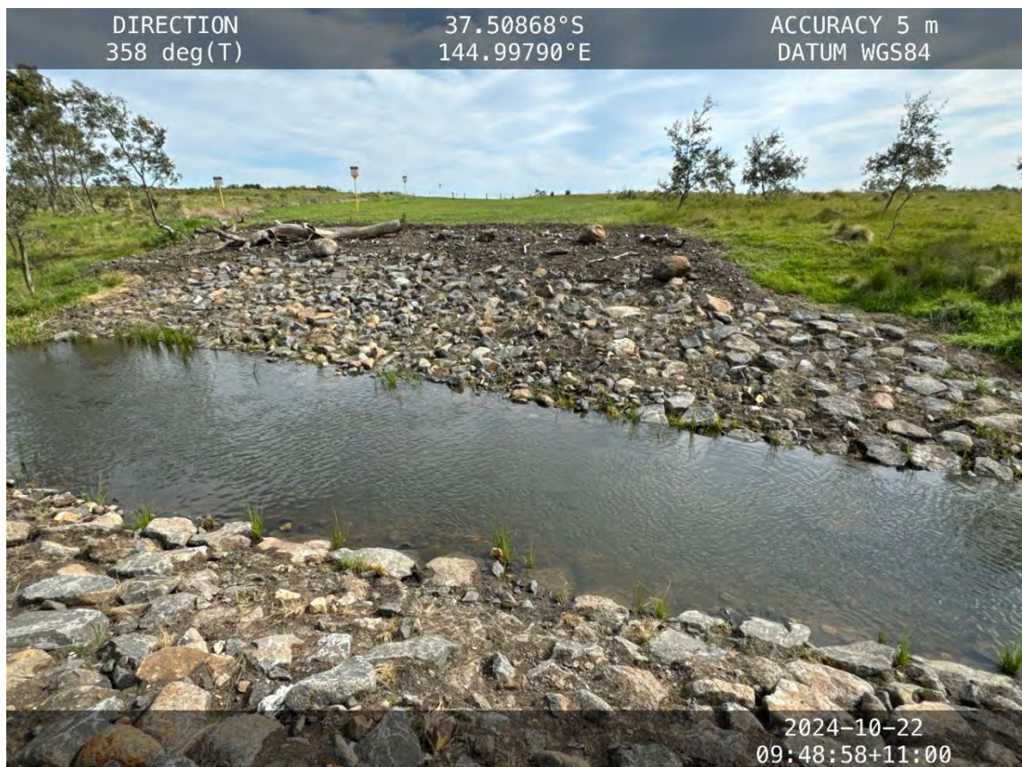
KP 42 Merri Creek – pipeline right-of-way with bank stabilisation, tubestock growth and exposed rock.
