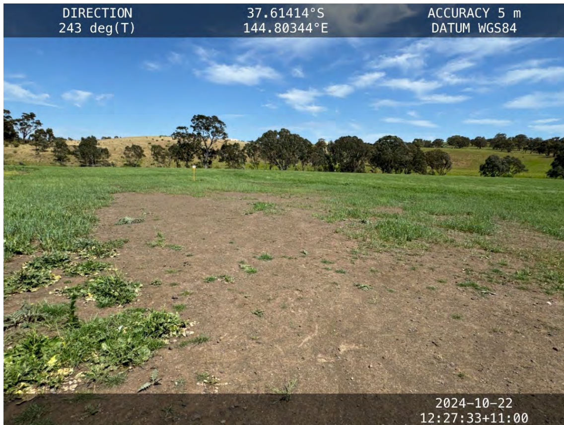
KP 16.8 Deep Creek – patch of bare soil at former HDD pad, tank and pit site surrounded by rehabilitated pasture.
