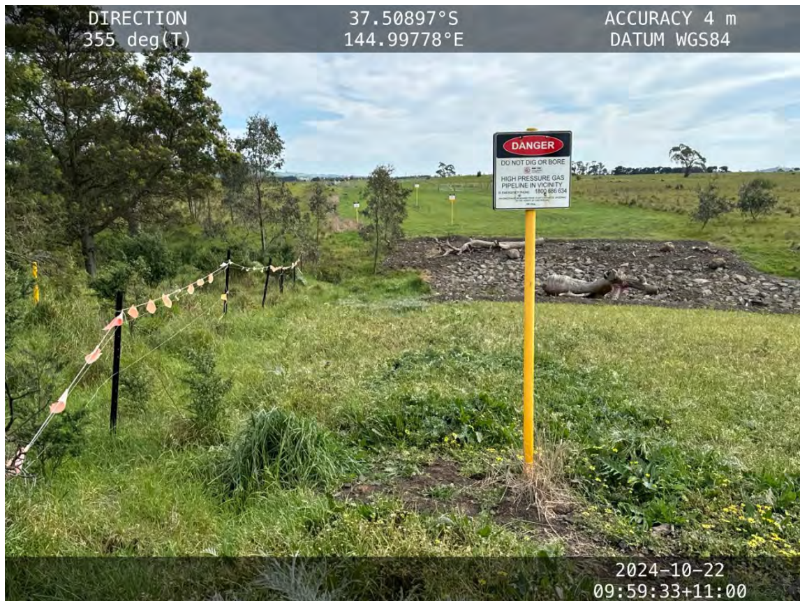
KP 42 Merri Creek – Pipeline marker and pipeline right-of-way border with vegetation growth.
