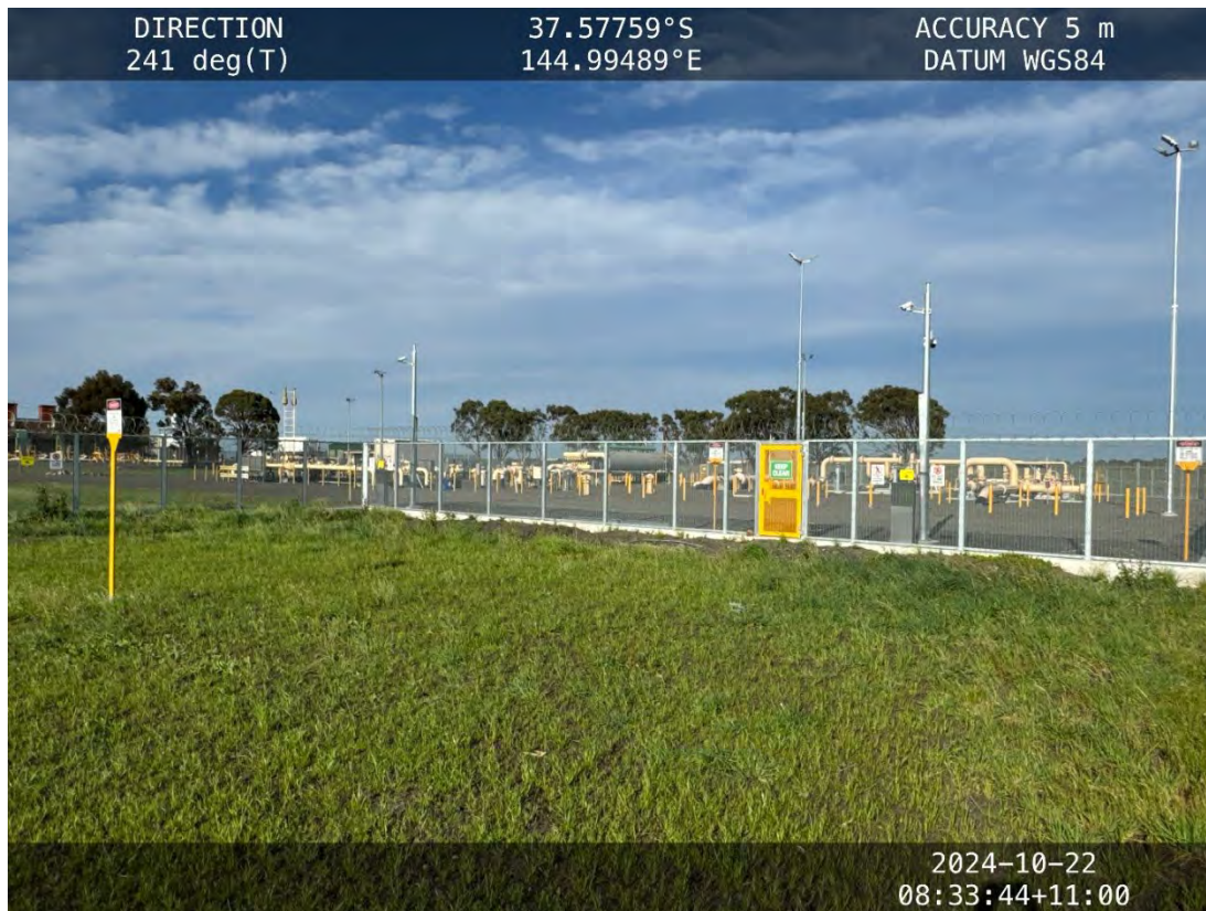
KP50 Wollert Compressor Station – rehabilitation surrounding the perimeter of the compressor station with pipeline marker.
