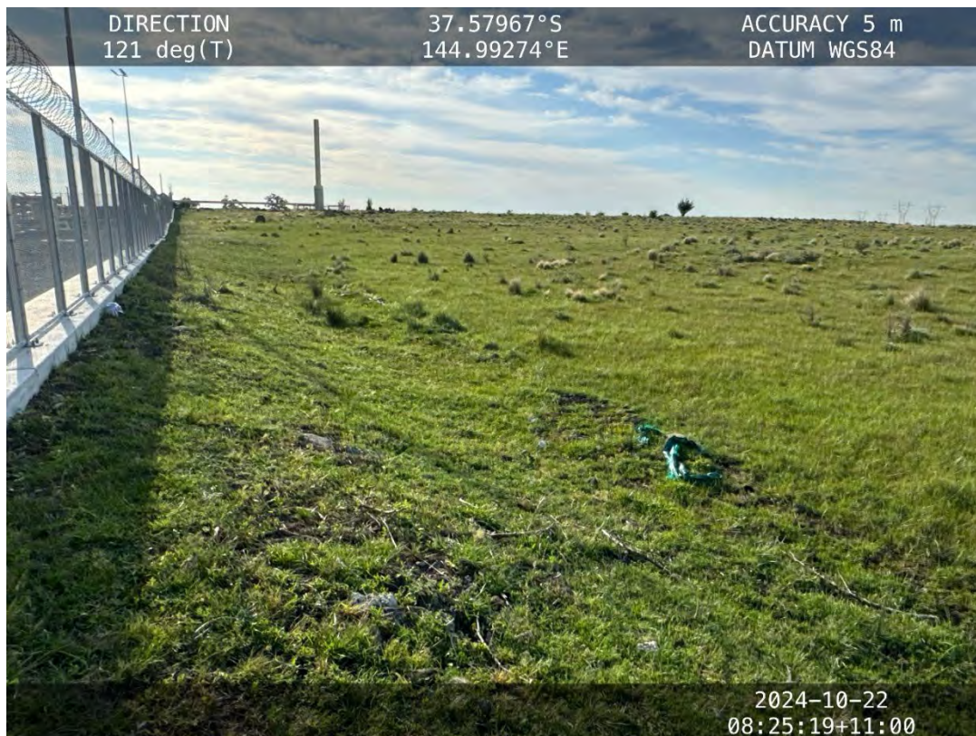
KP50 Wollert Compressor Station – stable and flat land surrounding the batters with remains of sediment fencing.
