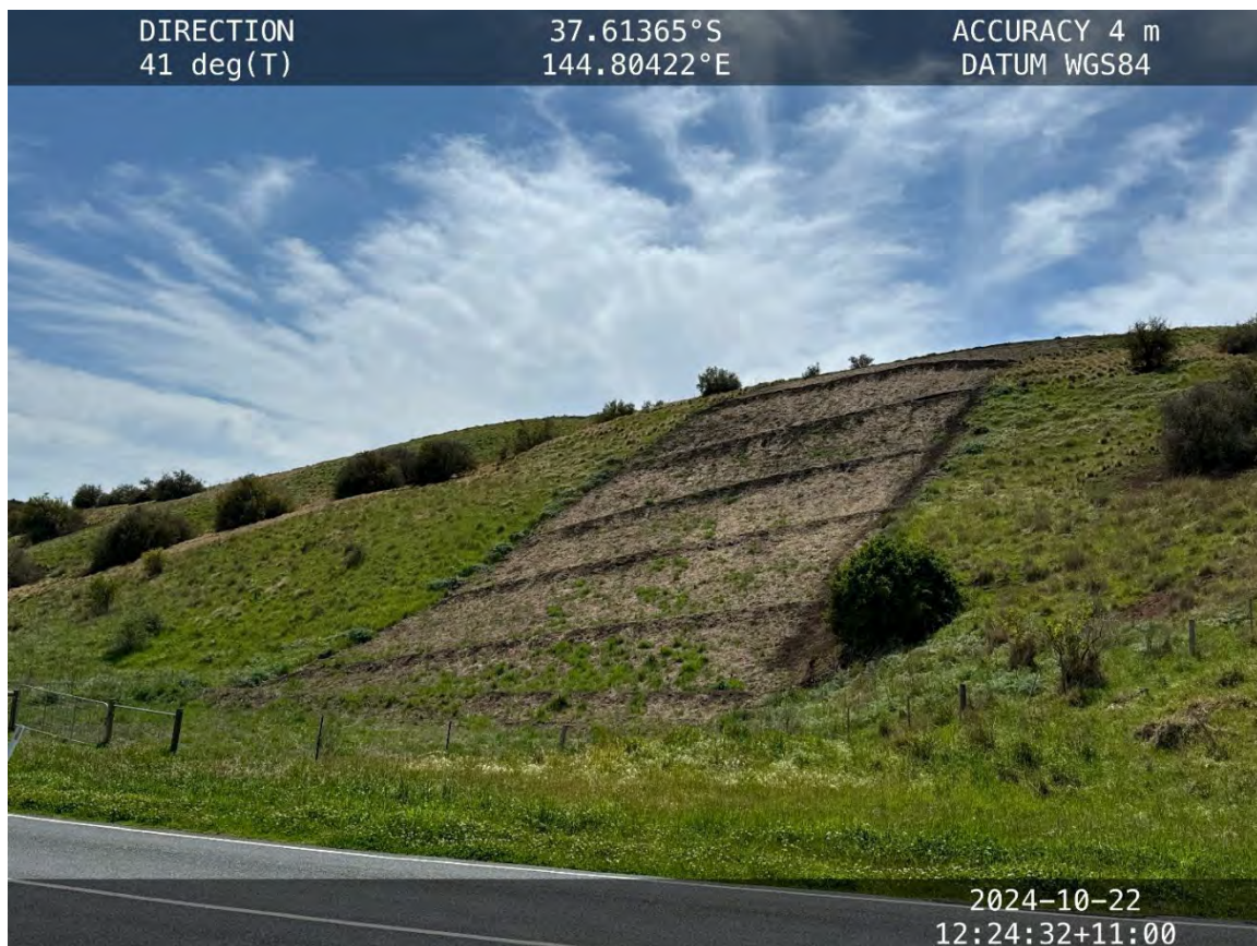
KP 16.8 Deep Creek – berms and vegetation growth upslope.
