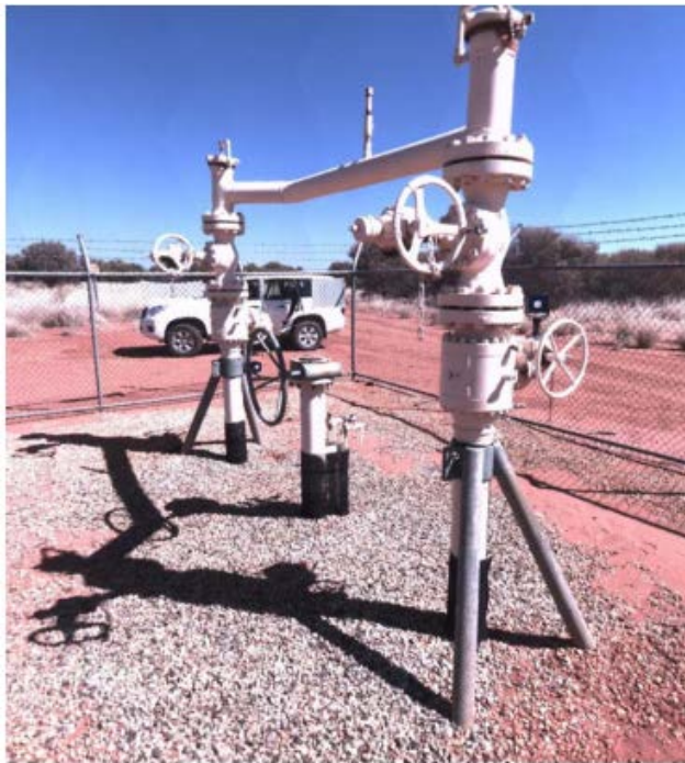
Figure 2-8: Typical Mainline Valve Station
