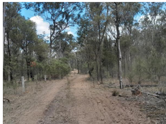
Figure 8-2 Graded access track / fire break
