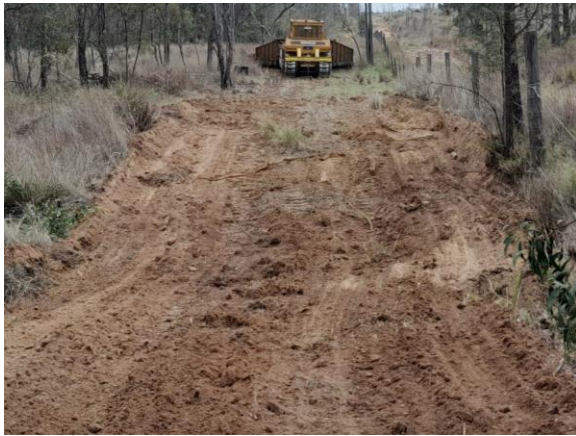
Figure 9-3 Graded access track / fire break
