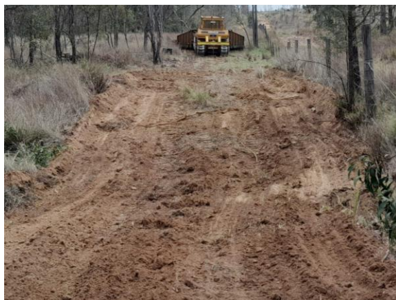
Figure 8-1 Graded access track / fire break
