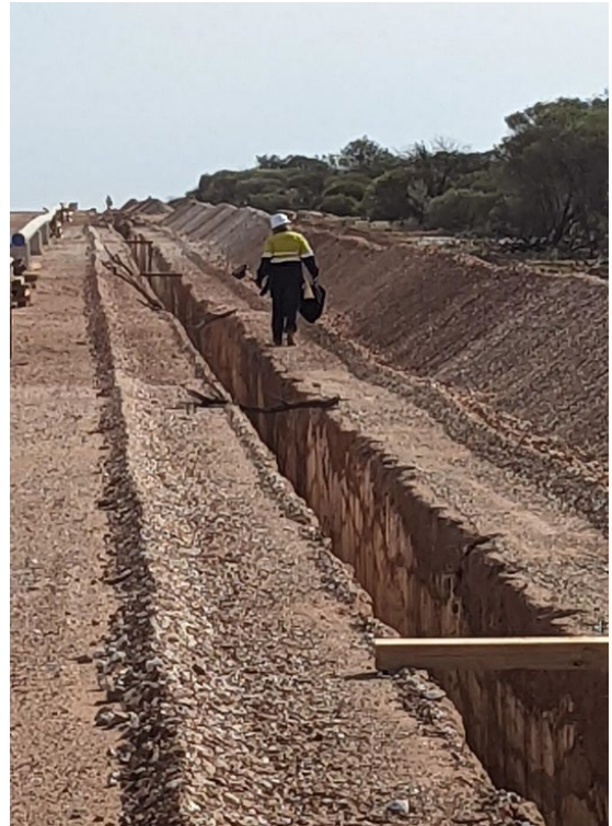
Plate 6. Trench Inspections – up to 10km each twice per day
