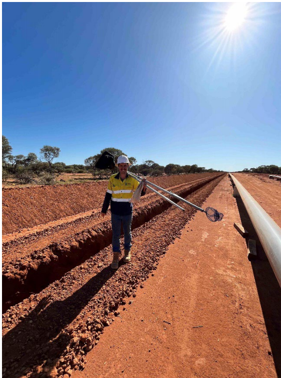
Plate 1: Trench Inspection Equipment
